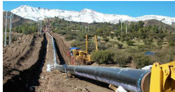
COPPER CONCENTRATE SLURRY PIPELINE 2
