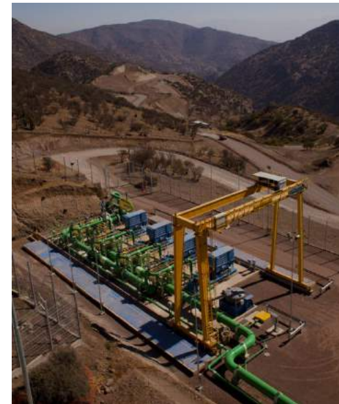
CONCENTRATE PIPELINE PUMP STATION 2
