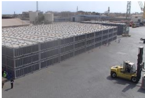
BULK CONTAINER LAYDOWN YARD
